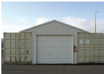
11. Conex boxes left over from construction were "married" with a common roof and standard garage-door access
