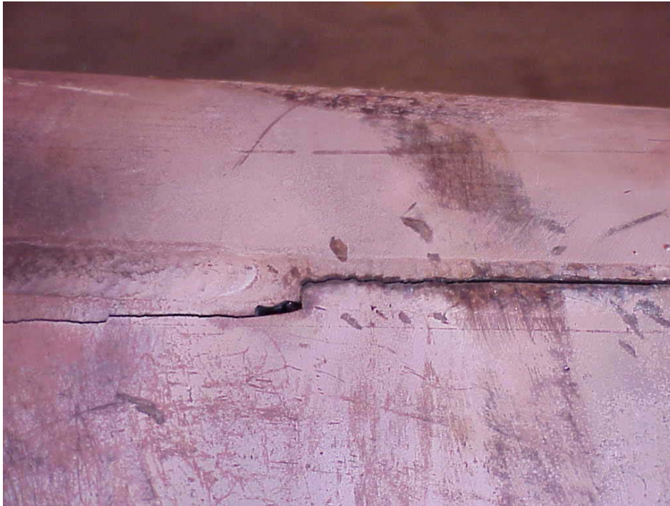
Figure 12.14: Weld Defects in Thermo Compressor
